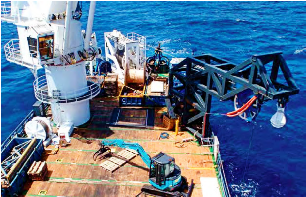
Dynlce Warp on drum winch, with large diameter sheave, aboard MV Seabed Worker
